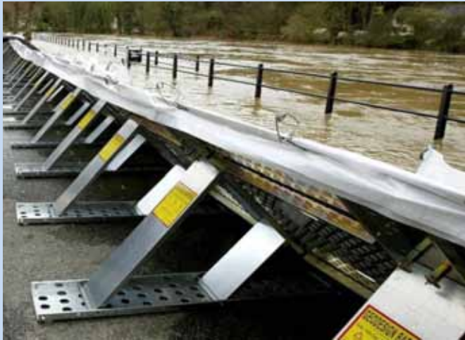
Flood Pathway Management: Temporary Flood Barriers
